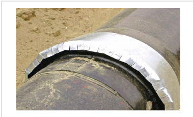
HDD metal protection cone for DIREXIONAL Universal Ve pipes
