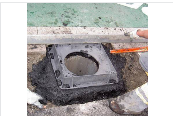
3- Upgrade of the frame.
