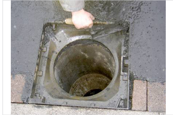
5- Cleaning of the seatings
