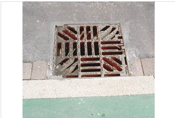
6- Grating in place.
