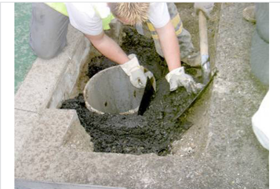
1- Implementation of the sealing product - PVC pipe
