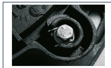
PAMTIGHT manhole covers - Anti-rotation clips
