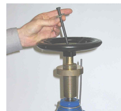
8- Installation of the handwheel and its fixing.
