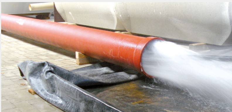
High pressure cleaning (120 bar)
