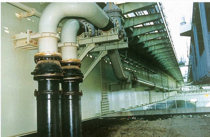
GEOFLEX® single ball joint DN 400 Overhead traverse in pipe gallery
