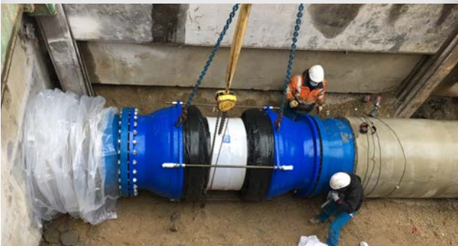
Laid at inlet/outlet of valve chambers
