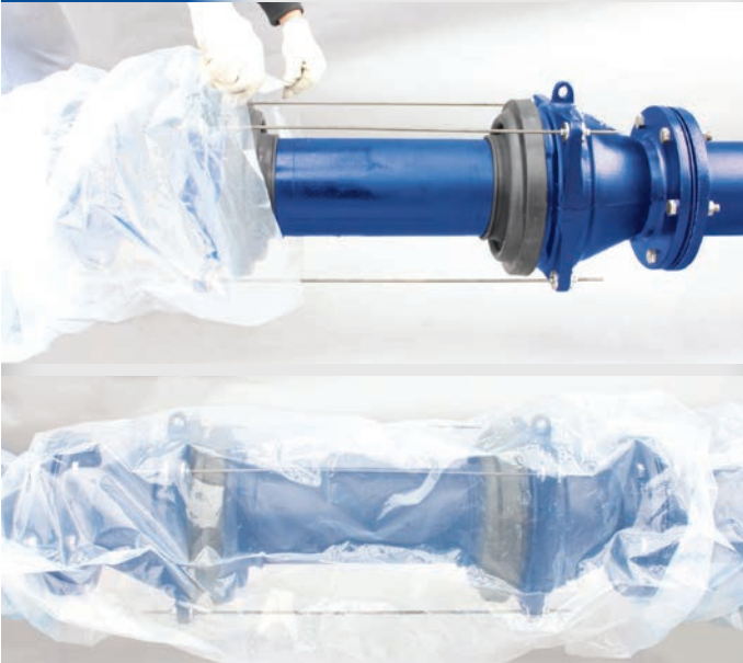
Install the polyethylene sleeve with the rods.
