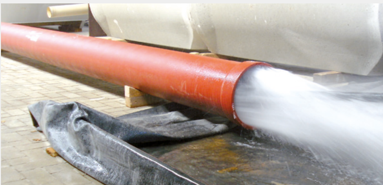
High pressure cleaning (120 bar)
