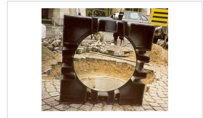
Manhole cover PAMREX 600 - D400 class - Installation of the manhole cover with apparent frame
