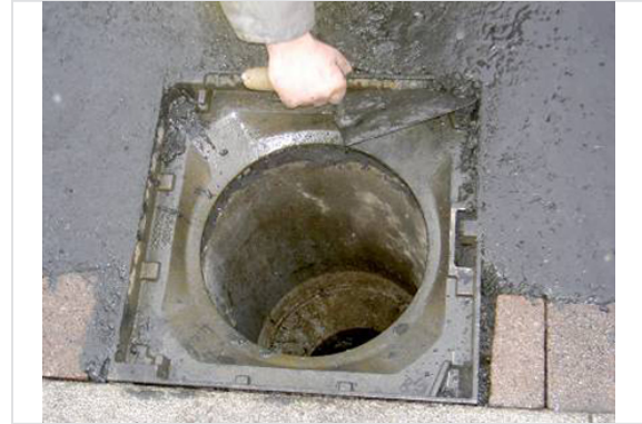
5- Cleaning of the seatings
