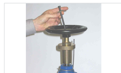
8- Installation of the handwheel and its fixing.
