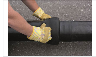
5- Slide the sleeve over the socket to protect the joint.
